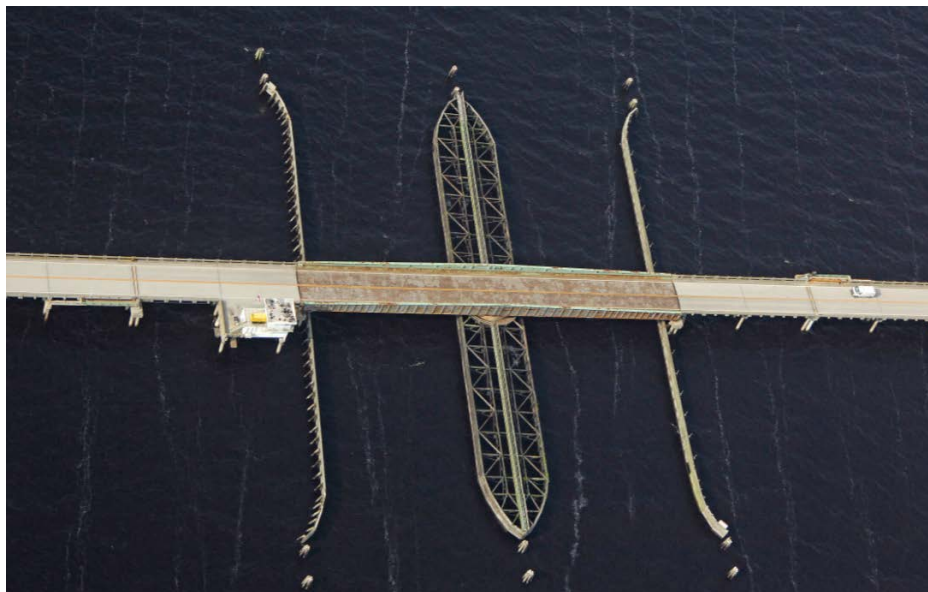
Figure 2: View of Existing Bridge
